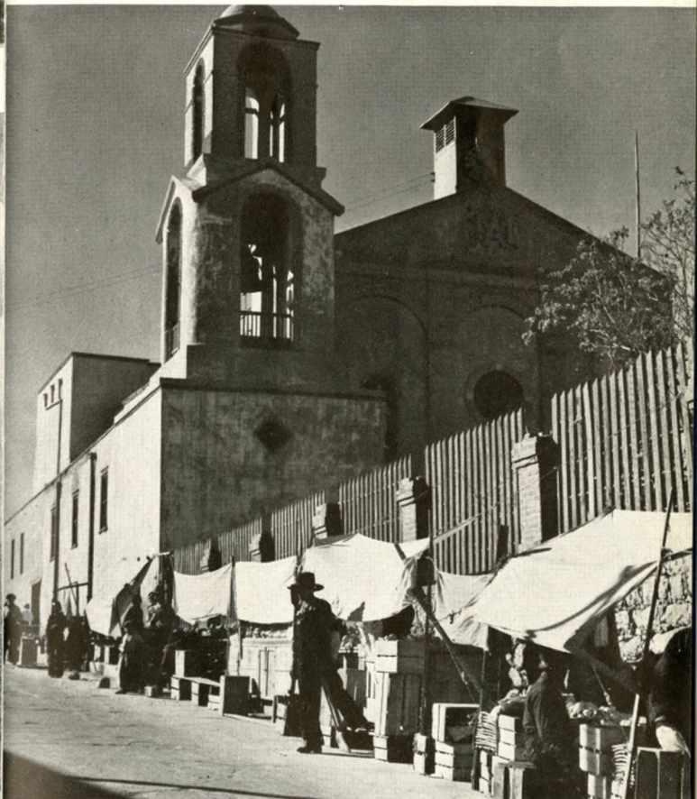
Vendors line the walks approaching old Guadalupe Mission in Juarez. The church was founded in 1659 and has adobe walls 56 inches thick.
