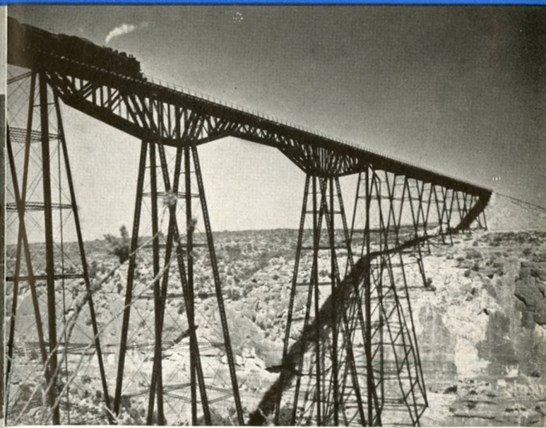
Tracks were practically laid in the air here. A Sunset Route train crosses the Pecos River Bridge en route from El Paso to San Antonio.
