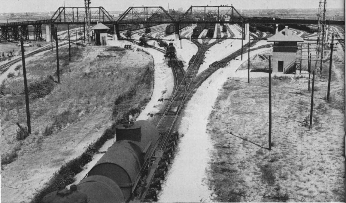
Gravity classification "hump" yards at Lincoln (above) and Galesburg expedite the movement of freight cars through these transportation hubs.
