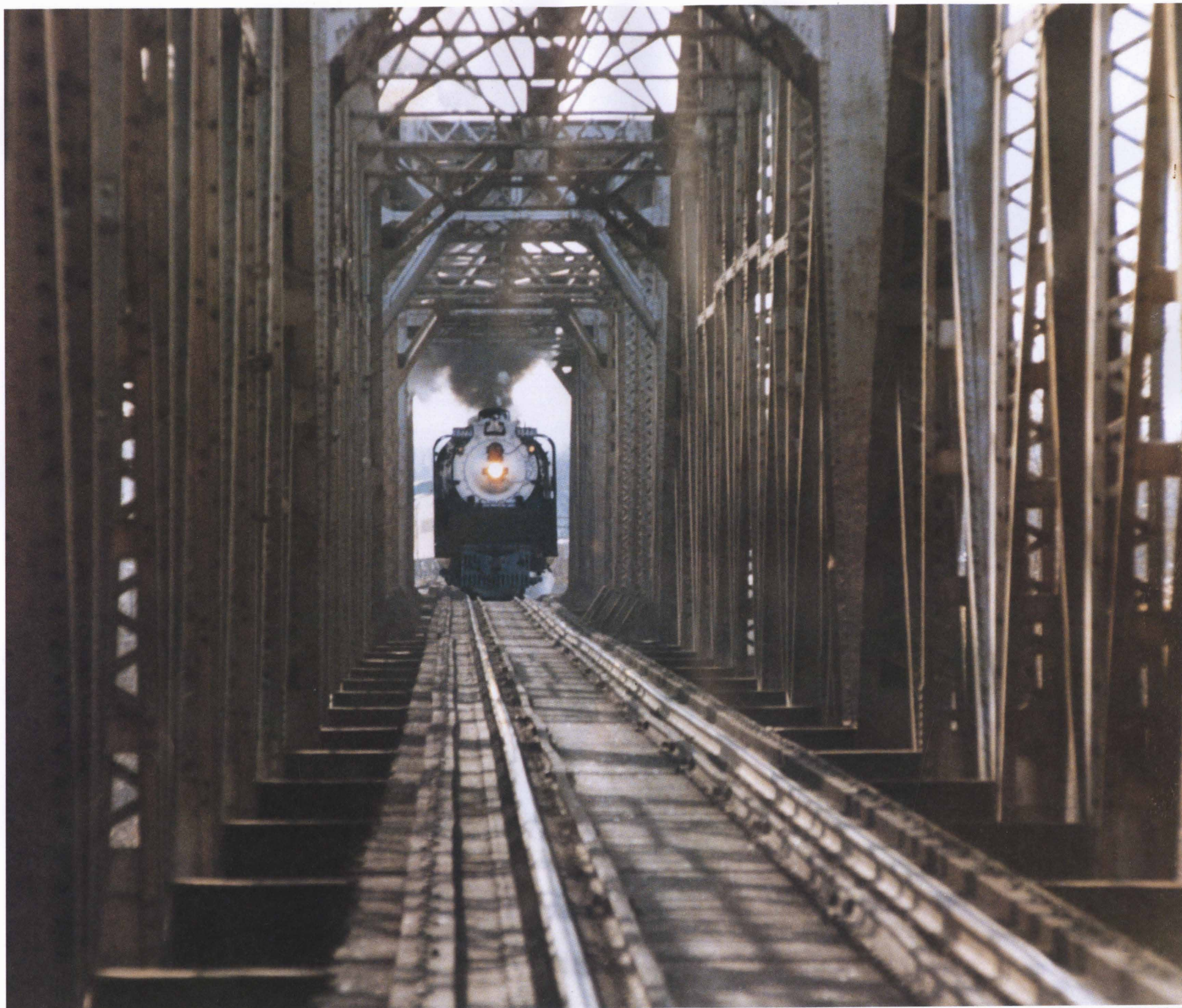
RED RIVER BRIDGE, DENISON, TEXAS
