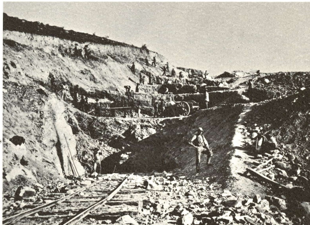
Hacking a cut out of solid rock UP graders had only picks and shovels, black powder and two-wheeled carts to work with.
