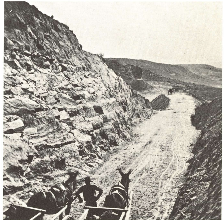
Far ahead of the tracklayers worked the graders, here shown making a cut through solid rock in Wyoming.
