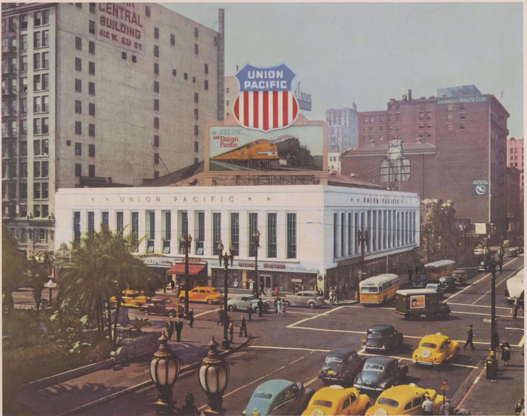
UNION PACIFIC BUILDING, WEST SIXTH AND SOUTH OLIVE STS., LOS ANGELES, CALIFORNIA
