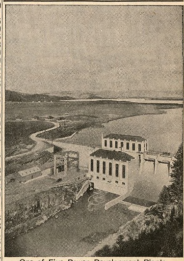
One of Five Power Development Plants on Historic Bear River, Utah
