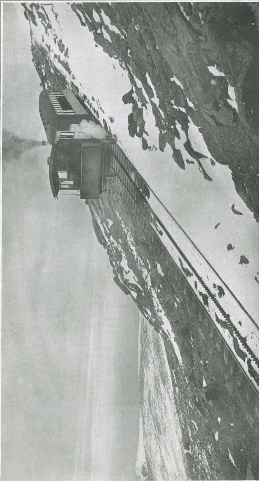
A Cog Road train climbing to the summit of Pike's Peak, the highest mountain in America whose summit is reached by a railroad. The Cog Road is unique in construction. From the Manitou station to the summit the road overcomes an elevation of 7,518 feet. The exact length is 47,992 feet and the average grade is 25 per cent. The roadbed is built of solid rock
