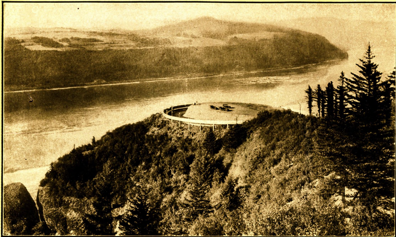
Crown Point , where the Columbia River Highway encircles the crest of Thor's Heights. For more than a mile beyond, between this point and the city of Portland, the Highway hangs on the edge of a cliff 925 feet high.
