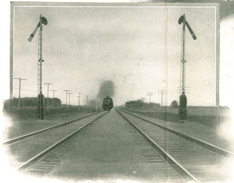
"Safety First," Double Track and Automatic Safety Signals on Union Pacific System
