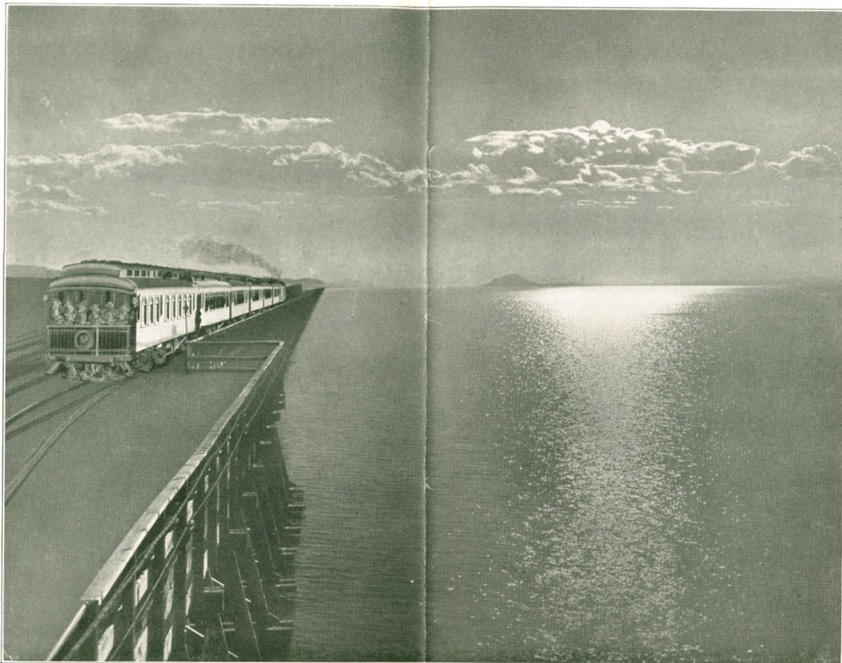
"Going to Sea by Rail" is a Novel Experience, where an $8,000,000 Causeway conducts the "Right-of-Way" across Great Salt Lake.
