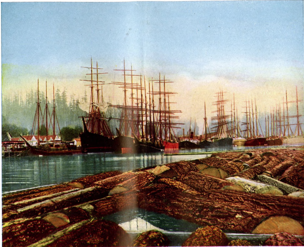
The sawmills of the Pacific Northwest turn out millions of dollars' worth of lumber every year
