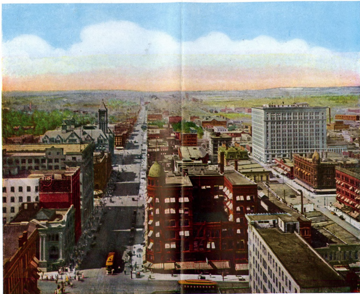
Omaha, Nebraska, with business district in foreground. Union Pacific Building, shown in upper right-hand corner, has Greater Floor Space than any other Structure in the City
