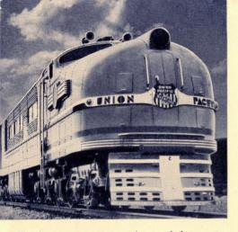
The locomotive consists of two of these units. Each is rated 2500 hp and can operate independently. The door in the "nose" opens into a passage to the operator's cab. One of the two headlights throws a beam straight upward as a warning signal when running in deep canyons through mountainous districts.
