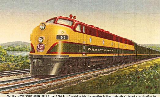
On the NEW SOUTHERN BELLE the 3,000 hp. Diesel-Electric locomotive is Electro-Motive's latest contribution to faster, more efficient railroading.
