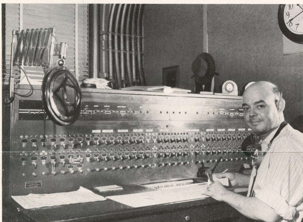
D. A. Benson operates one of Southern Pacific's Centralized Traffic Control systems. "C. T. C." gives dispatcher direct control of switches and signals governing proper movements of trains. The system, costing approximately $15,000 a mile, increases capacity of single track as much as 50 percent. S. P. is installing C. T. C. at critical points on the line.
