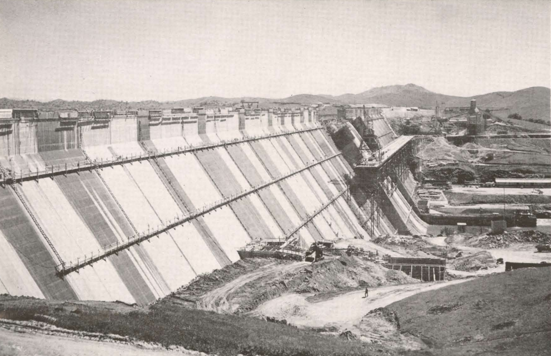
Friant Dam is second largest unit in Central Valley Project and fourth largest dam in the world. Twenty miles north of Fresno, it will control the San Joaquin River, creating a reservoir 15 miles long. Height of dam 320 feet; length 3,430 feet; volume 2,200,000 cu. yds.
