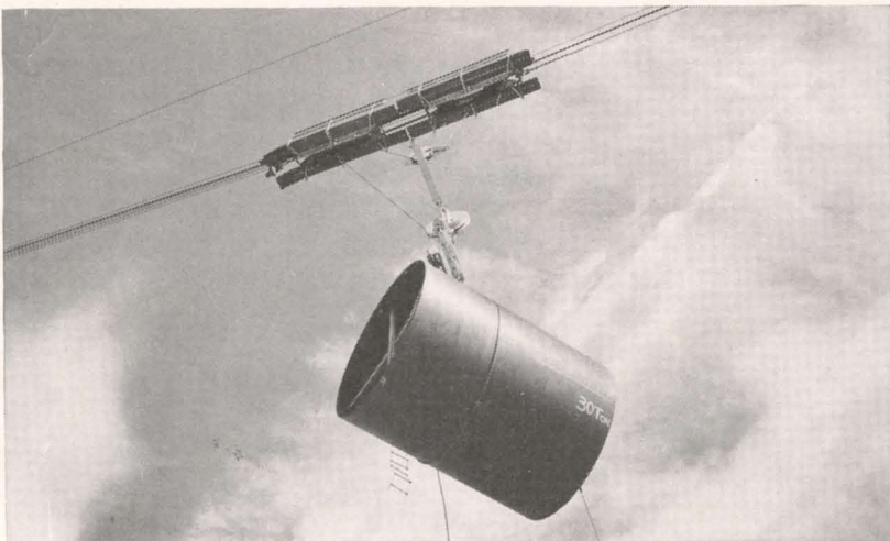
This little piece of pipe is 15 feet in diameter and weighs 30 tons! It is a section of one of the penstock pipes for the Shasta Dam powerhouse.
