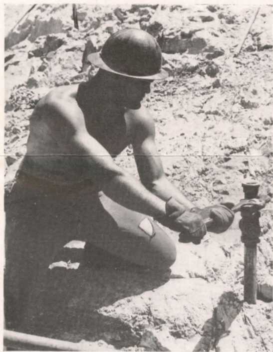
Pete Mercendetti connects a valve to a "grouting" pipe extending into the foundation of the damsite. All workers wear steel helmets.
