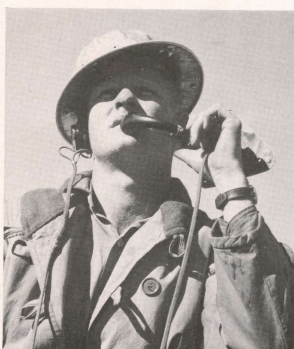
Cableway signalman on construction site uses telephone to direct operator in distant head tower.
