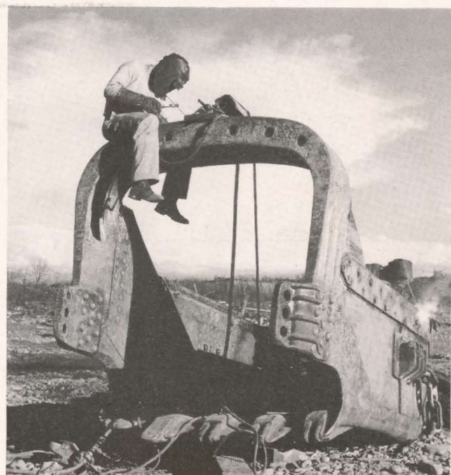
Looking like a mythical "man from Mars," this unidentified welder is repairing a giant bucket in the gravel pit.
