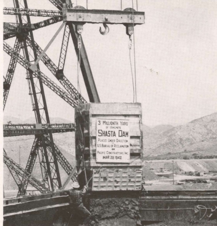
This picture records the halfway point in the construction of Shasta Dam—pouring of the three millionth cu. yd. of concrete, March 28. Pouring proceeds at rate of 200,000 cu. yds. a month.
