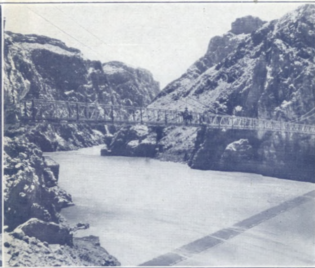
New suspension bridge across Colorado River near Phantom Ranch
