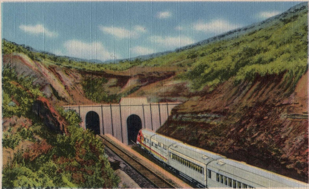
H-1561 RATON TUNNELS, BETWEEN TRINIDAD, COLORADO AND RATON, NEW MEXICO
