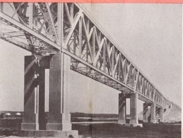
SAMSON OF THE CIMARRON —Typical of Rock Island progress in the improvement of its right-of-way is this huge span at Liberal, Kansas. More than 1,200 feet long and rising more than 100 feet above the river, the bridge shortened the old line 3.6 miles. Rock Island's continuous maintenance program is eliminating curves, leveling roadbed, increasing traffic speed.
