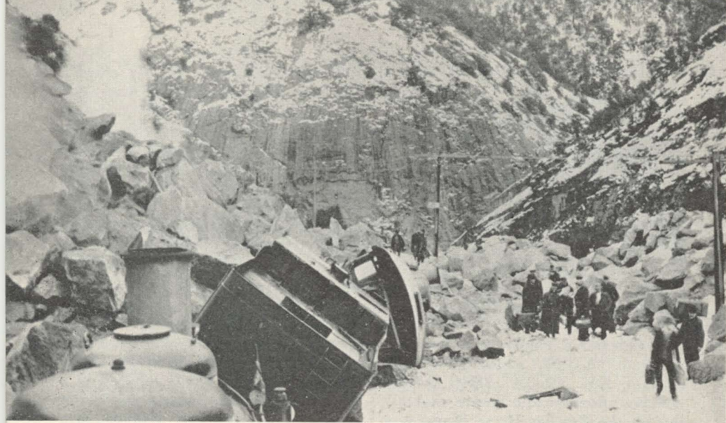
The Canyon was not tamed with the driving of the Last Spike. Until slopes had been scaled back and insecure boulders minimized, incidents like that above at M. P. 246 made the locomotive engineer's job similar to the airline pilot's of today.
