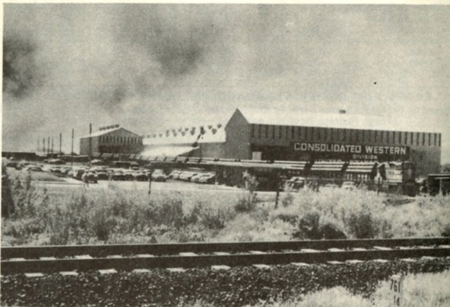
Consolidated Western Division of U. S. Steel Corporation manufactures expanded steel pipe for industry in this new, modern plant at Provo, Utah, on Rio Grande's main line.
