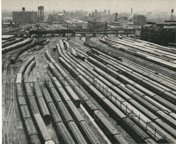
Extensive improvements have been made to the passenger coach yard at Chicago where Pennsylvania's daily fleet of eastbound trains are cleaned, inspected and assembled.
