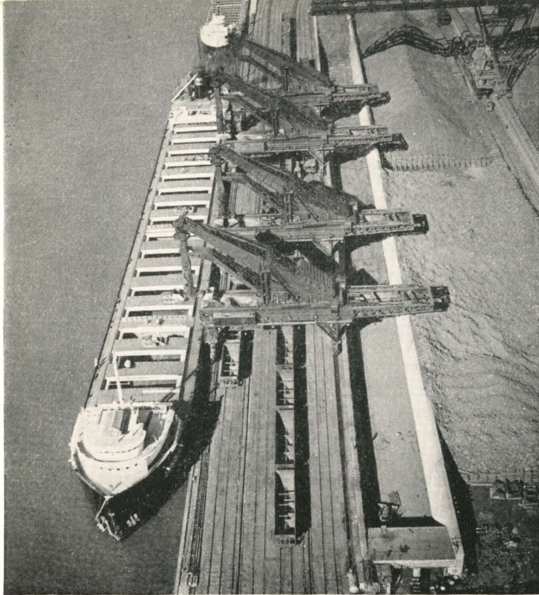
Rail loadings of ore at Great Lake ports set new records in 1953. Above, the Pennsylvania's modern ore pier at Cleveland, Ohio, one of the largest docks on the lakes.
