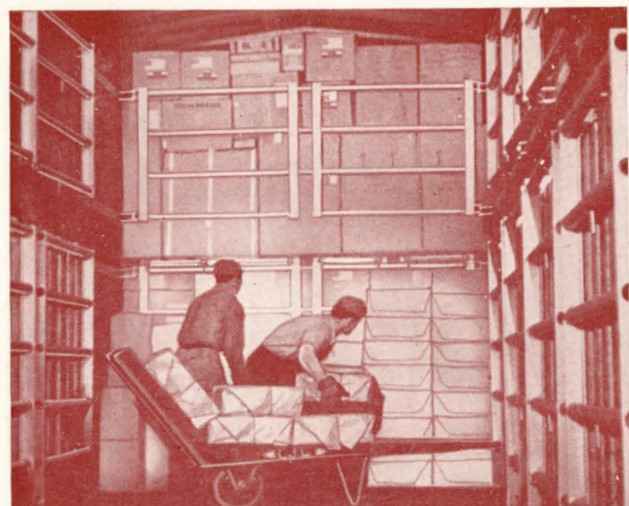
INTERIOR of new merchandise car showing new racks to safeguard shipments against damage.
