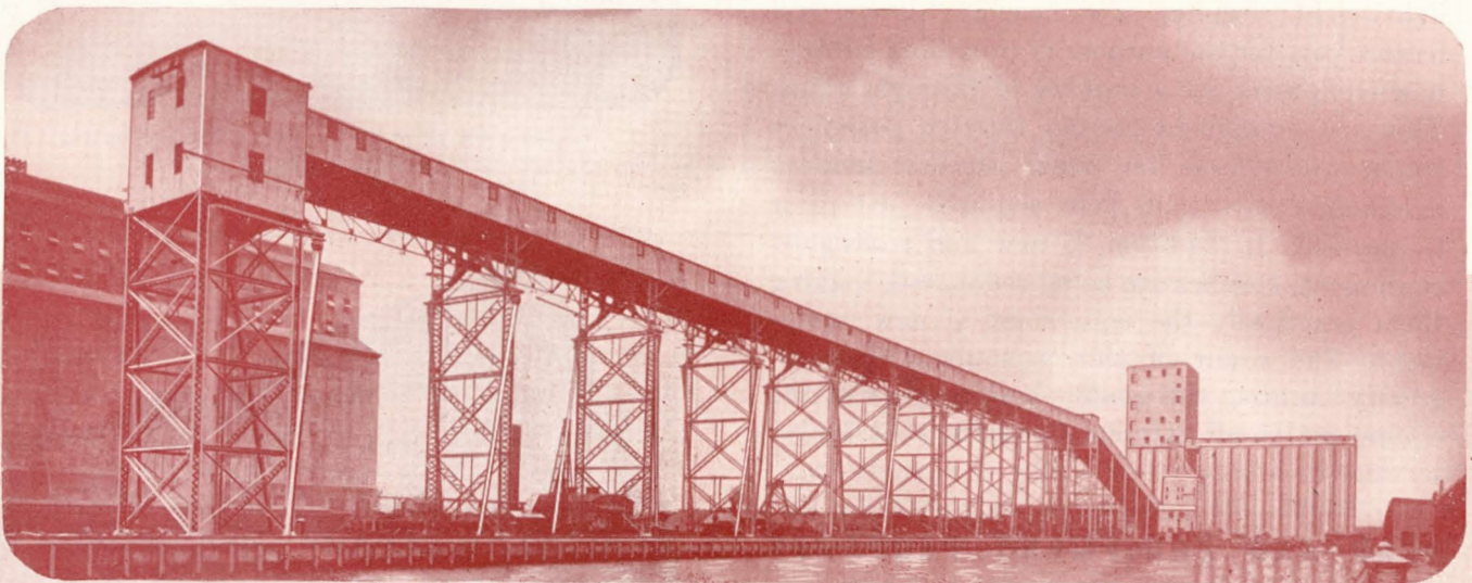
GRAIN FOR HUNGRY EUROPE moves up this great conveyor to be loaded into ships from the elevator in the background. Pennsylvania Railroad maintains great installations similar to this at principal Atlantic seaboard ports.
