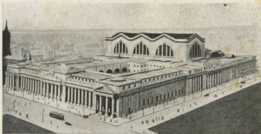
Pennsylvania Station, New York City
