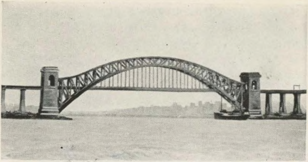
Hell Gate Bridge
