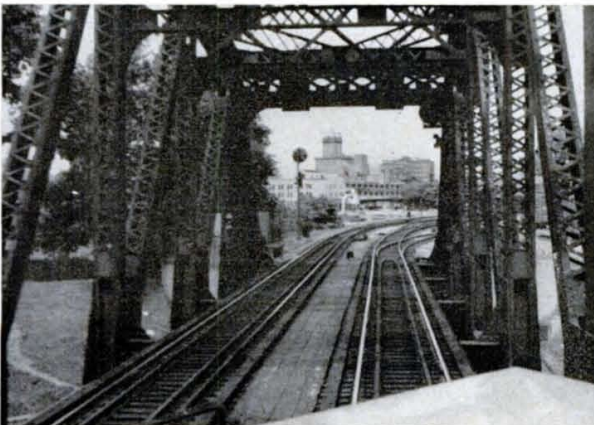
The Xplorer noses onto a truss bridge. Cleveland-Cincinnati run pits the new train against auto, bus and airline competition.
