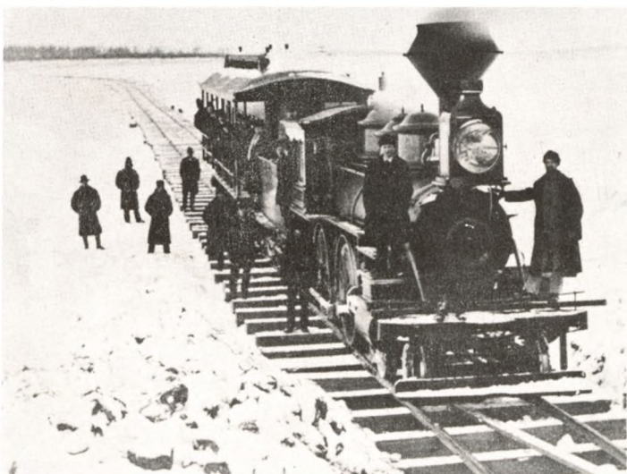
RAILS ON ICE allowed Northern Pacific trains to cross Missouri River from Bismarck to Mandan during winters of 1879-82.
