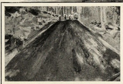
Track Grading. End of a Dump.
