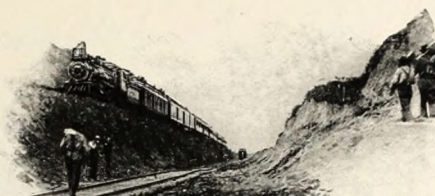
Reducing a Grade. Last Train over OLD Main Line. New Track Seen in Cut before Leveling, etc.
