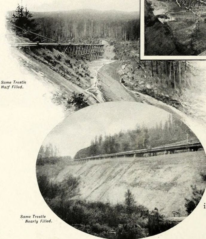
Sluicing Down the Mountains and filling Trestle by Means of Giant Nozzles.
