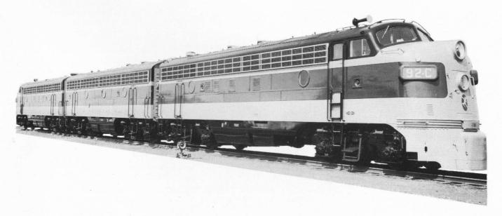
DIESEL-ELECTRIC Passenger Locomotive No. 92 (Model Fp-7)—Built in 1950 by Electro-Motive Division, General Motors Corporation. This 3-unit passenger locomotive is rated at 4500 horse power. Each of three Diesel engines drives an electric generator which produces 1500 horse power at full load speed, 800 r.p.m. Traction motors are geared to 40-inch driving wheels.
