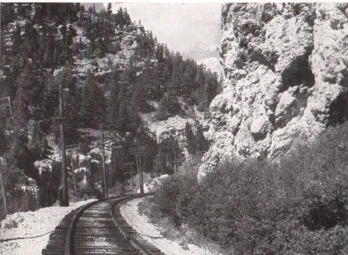
Over the Continental Divide with electric power. Substations reduce the voltage from 100,000 to 3,000 and change it from A.C. to D.C. before sending it out over the trolleys.
