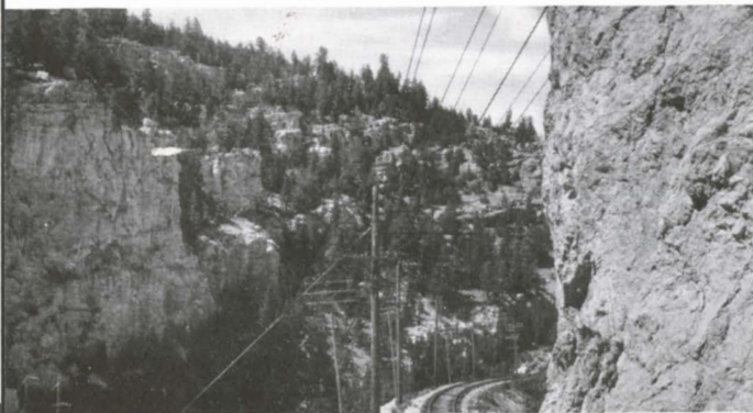
Over the Continental Divide with electric power. Substations reduce the voltage from 100,000 to 3,000 and change it from A.C. to D.C. before sending it out over the trolleys.
