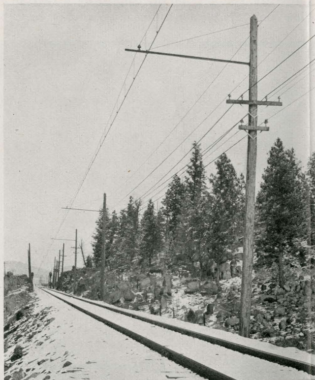
TANGENT BRACKET TROLLEY CONSTRUCTION
