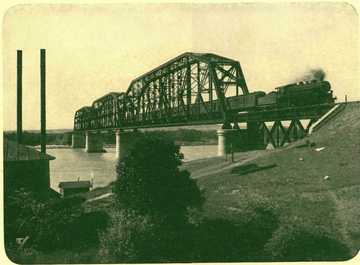
Steel Bridge, Missouri River, Mobridge, S. D.
