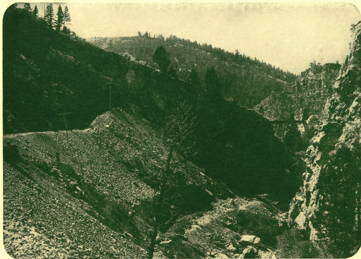
Eagles' Nest Tunnel, Montana Canyon
