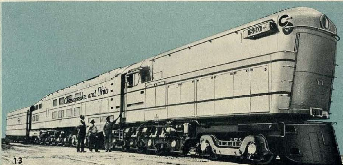
One of the three steam turbine electric locomotives of the Chesapeake & Ohio Railway.
