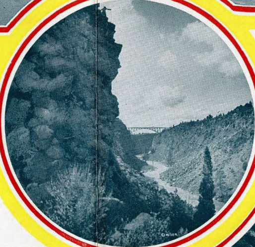
Crooked River Bridge, 320 ft. high © Kiser
