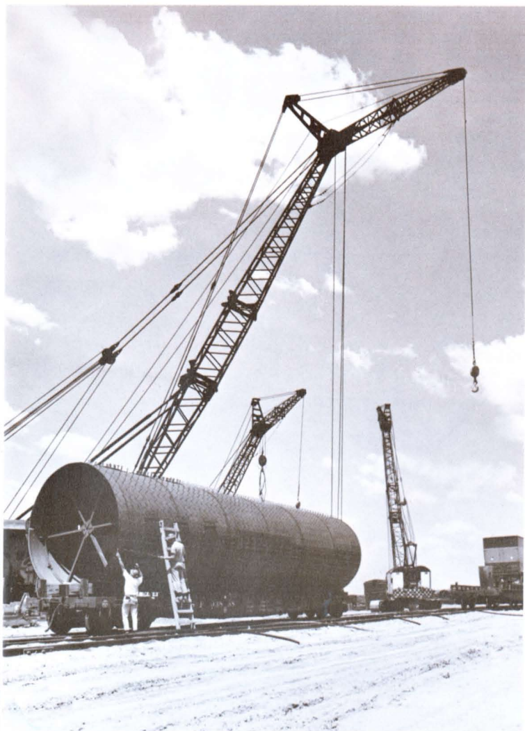
Launch tube section for a Minuteman missile arrives by rail at bustling Bethlehem steel yard in Minot. These and other steel components were moved to widespread launch and control sites by GN truck.
