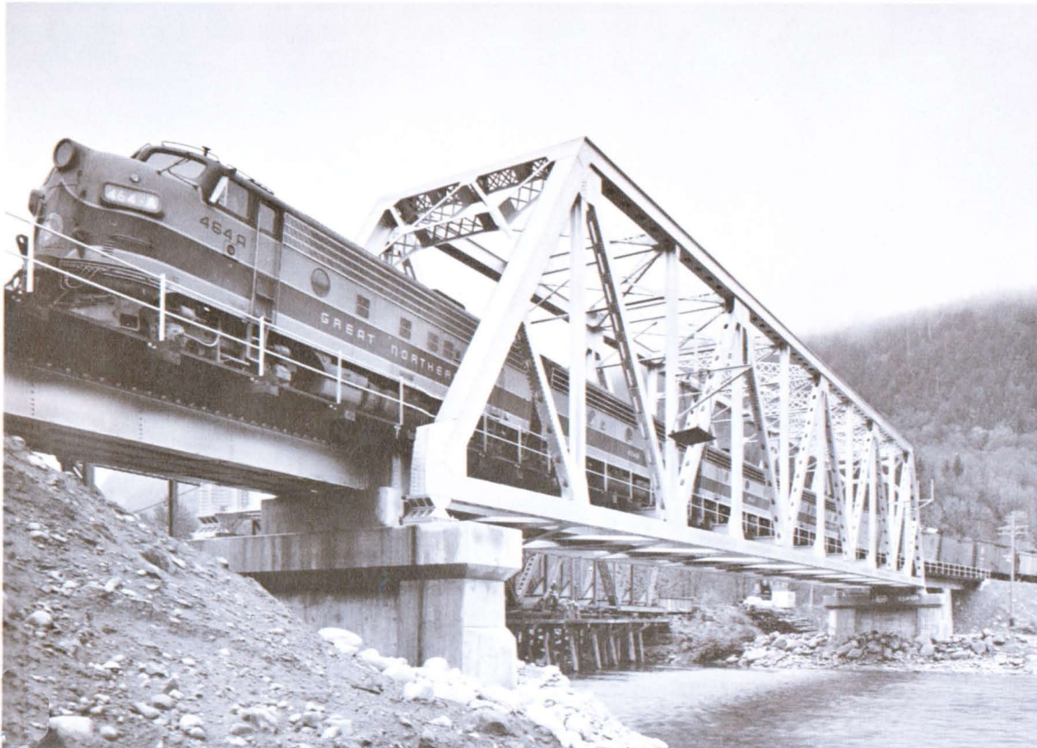
This new 225-foot steel truss span across the North Fork of the Skykomish River is part of a major relocation project in the Cascade Mountains. Partially dismantled old bridge can be seen in distance.
