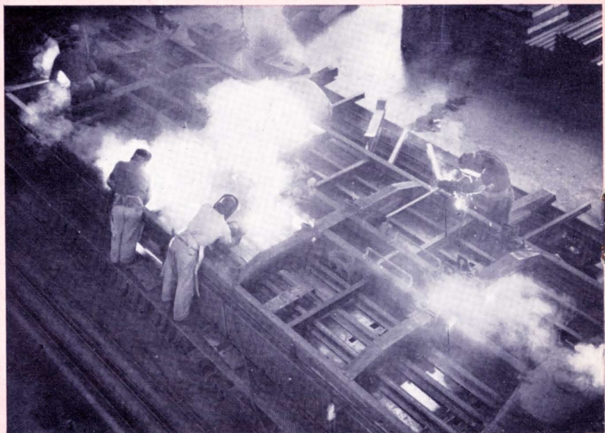
Welding Under Frames
