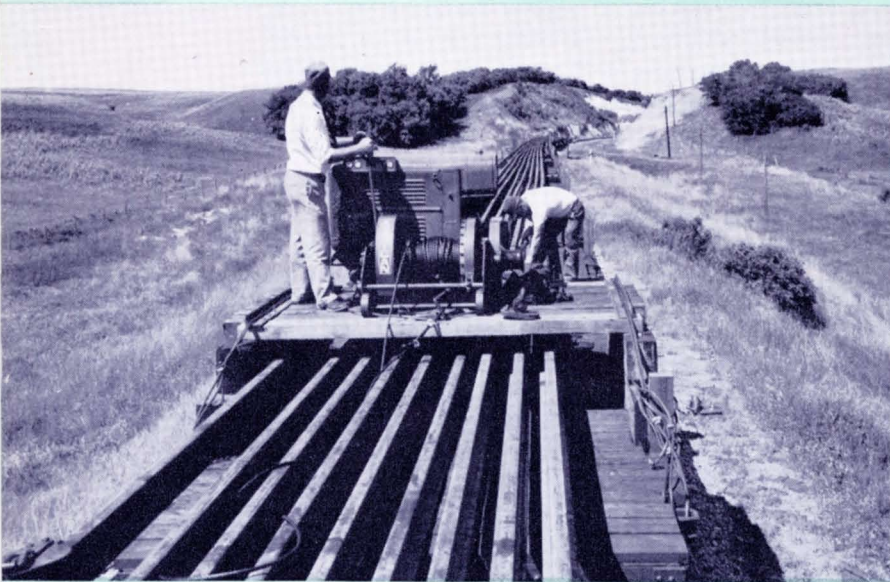
UNLOADING THREE MILES OF WELDED RAIL PRIOR TO PLACING IN TRACK.
