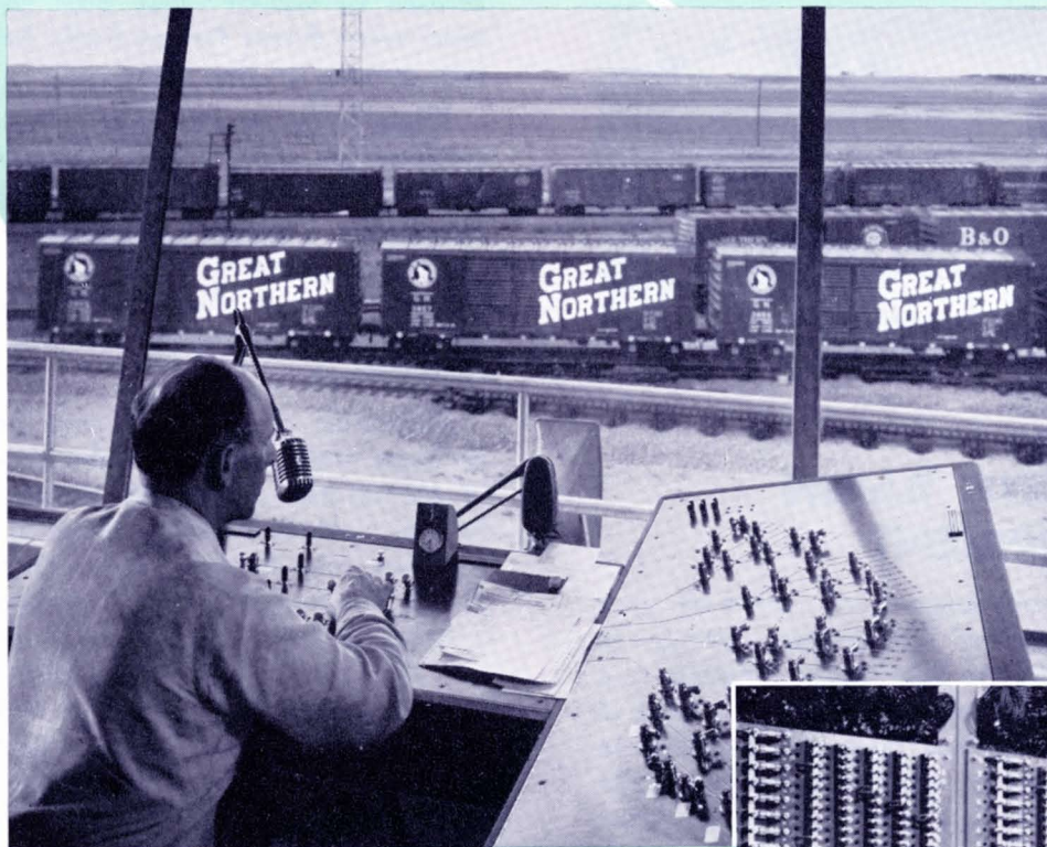
5 An Operator Checks and Supervises Car Movement by Gravity into the Proper Track.
