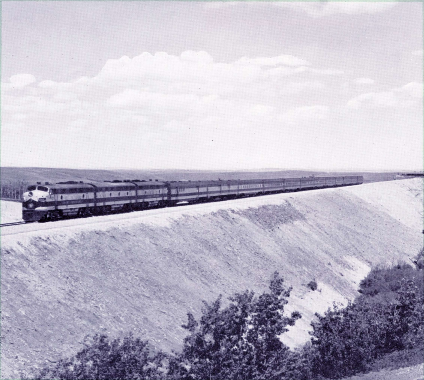
FIRST TRAIN OVER NEW 1.2 MILE FILL - MAXIMUM HEIGHT 65 FEET - OLD LINE IN FOREGROUND
