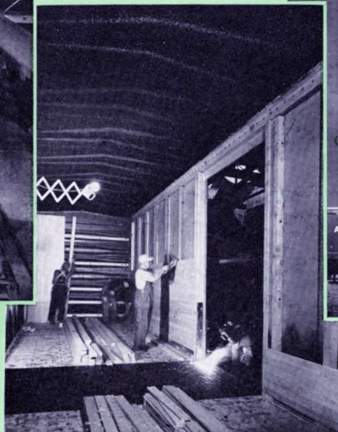
Installing Lumber Lining
