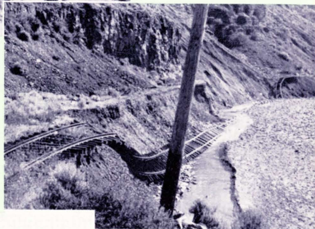
Mansfield Branch, Central Washington, damaged by three separate flash floods for 27 miles.
