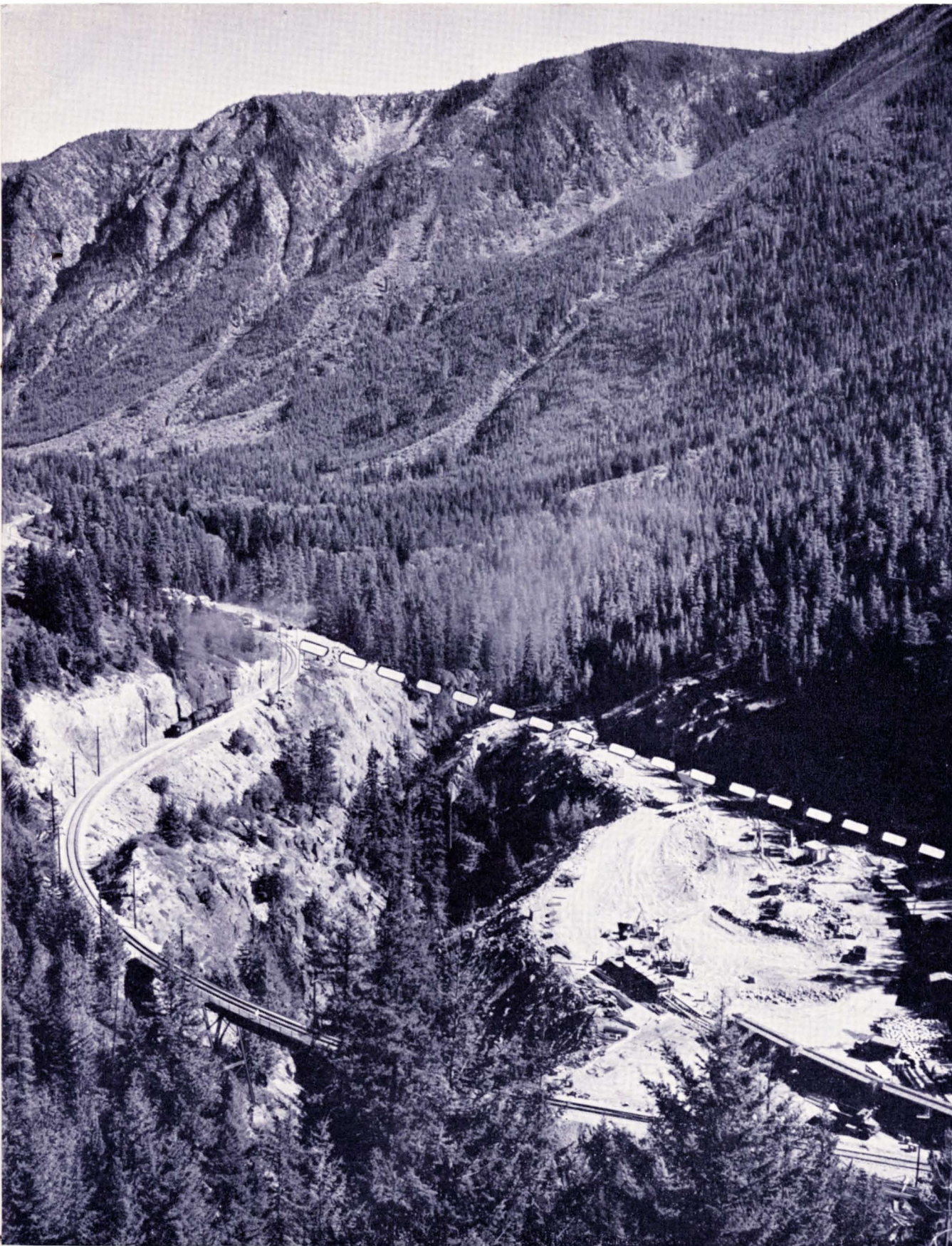
$1,000,000 line relocation on East slope of Cascade Mountains shown by heavy dashed line. Eliminates five sharp curves. Will be completed in Spring of 1949.
