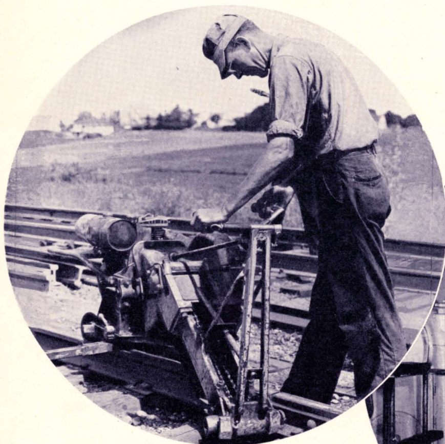
TRACK MAN TIGHTENING BOLTS BY MACHINE.
