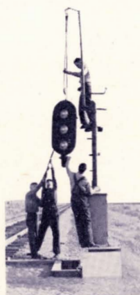
AUTOMATIC BLOCK SIGNALS, MINNEAPOLIS TO ST. CLOUD, MINNESOTA.
