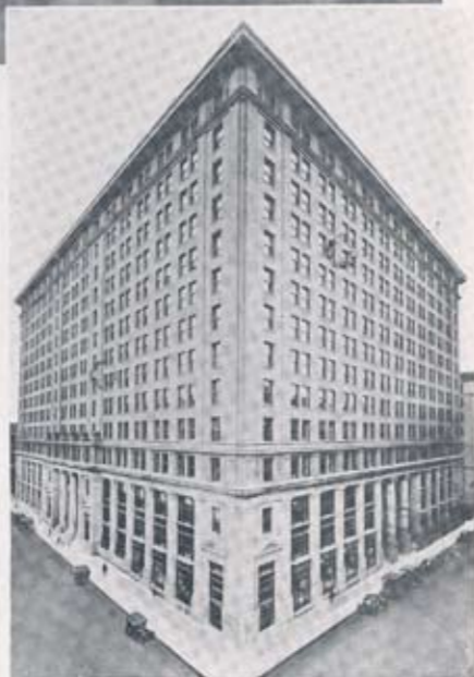
General Office Building, Great Northern Railway.
