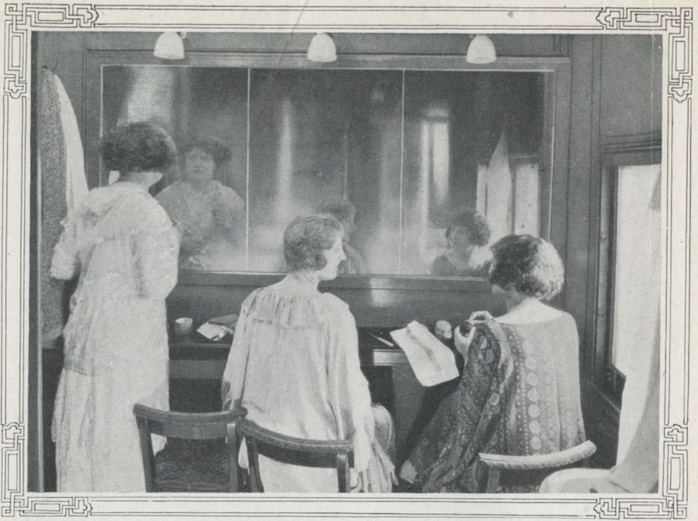
Women's Wash Room
