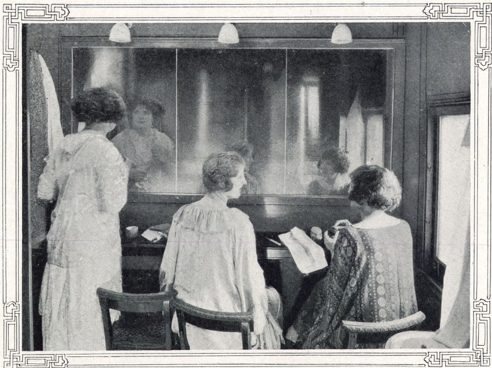
Women's Wash Room
