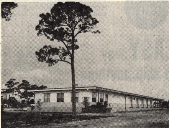
The new Freight Depot is equipped to efficiently handle a large volume of traffic.
