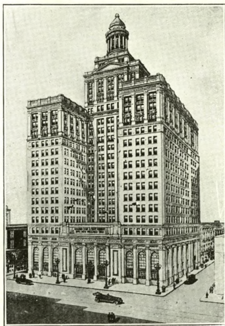
Hibernia Bank Building New Orleans Headquarters, Passenger and Freight Depts., I. C. R. R. 10th Floor
