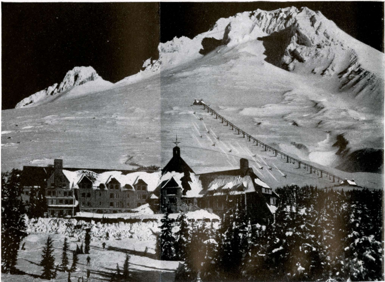
Timberline Lodge, mile-high, all-year resort on Mt. Hood, Oregon.
