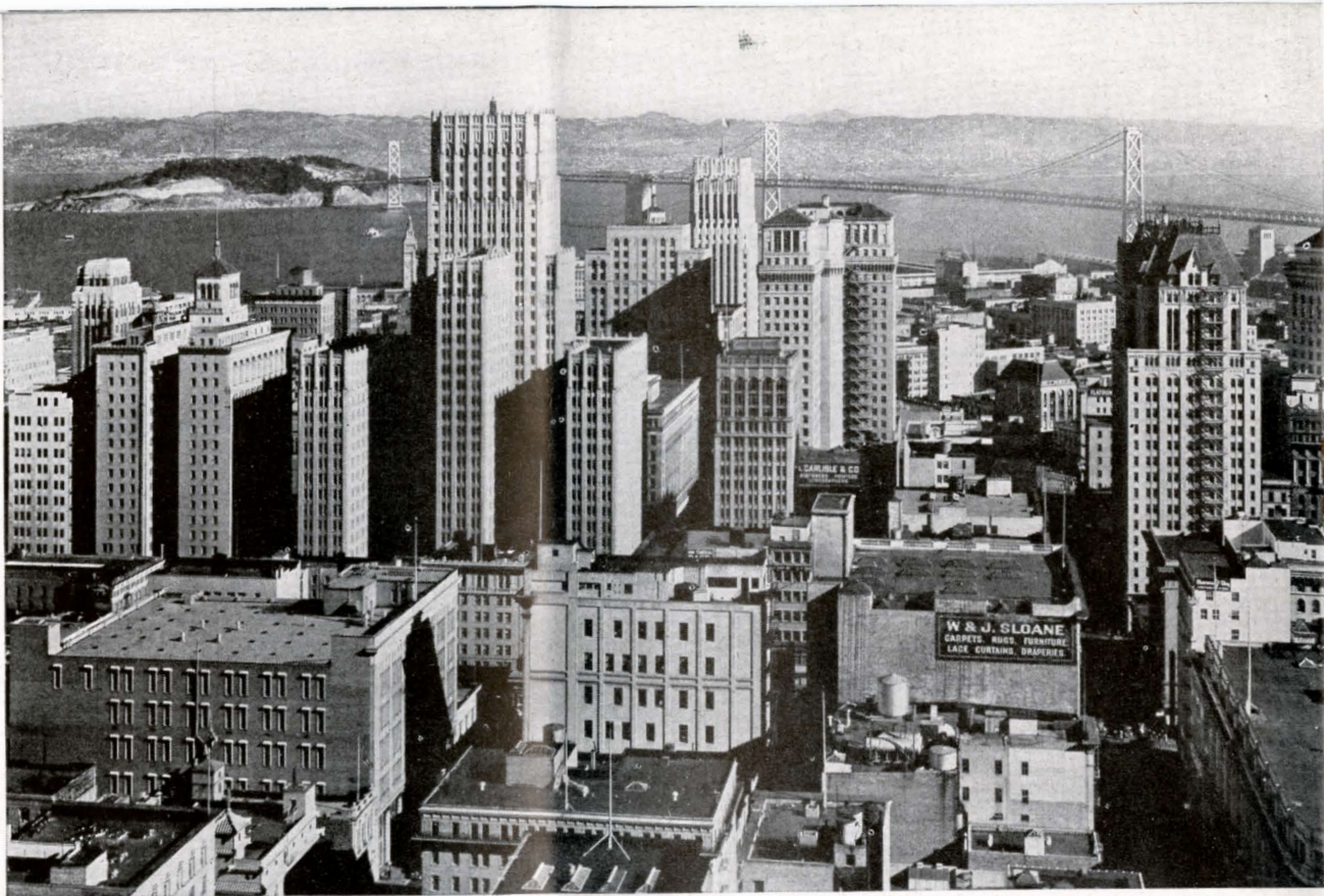
A portion of downtown San Francisco showing a section of the San Francisco-Oakland Bay Bridge
