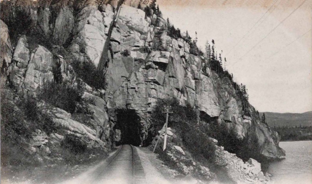
JACK FISH TUNNEL, LAKE SUPERIOR (LOOKING EAST). ON CANADIAN PACIFIC RAILWAY
