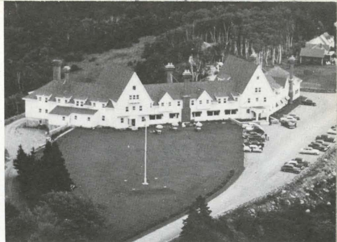
▲ Keltic Lodge—noted summer resort at Ingonish, N.S., is a typical retreat for the city dweller.
