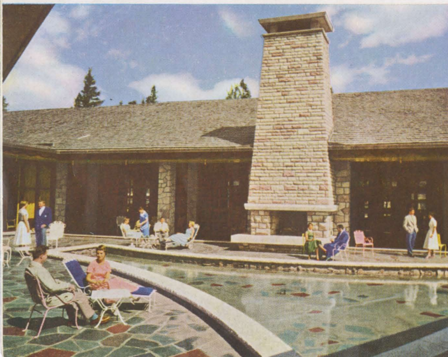
The patio, at the heart of the Central Building, is open to the sky.
